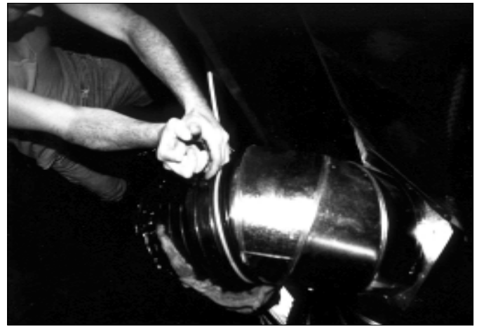
Heat crossover connection details: The inner liner is mechanically secured to the elbow with a zip tie. Note use of the appropriate strap tightening tool. Hand tightening doesn't work. The inner liner will be air-sealed to the elbow with tape. To complete the connection, the outer liner will be drawn up over the elbow to the V-box and mechanically fastened/strapped in place. V-box insulation should be installed and tape/sealed to close the V-box penetration through the belly fabric and the seal the V-box insulation to the outer liner of the flex duct. These seals keep Mickey Mouse from moving into the belly. Excess pieces of the outer liner with vapor barrier are acceptable materials for insulating the V-box.
